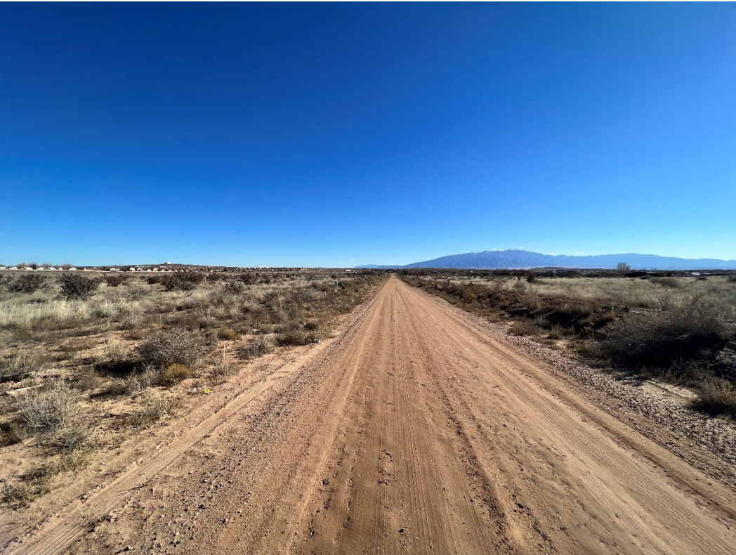
Photo 6: Bladed dirt road (facing east)
