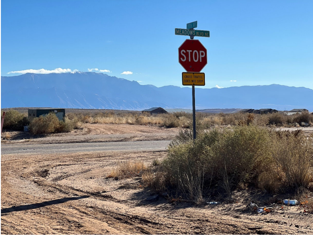
Photo 1: 28 th Avenue and Meadows Boulevard Intersection (facing southeast)
